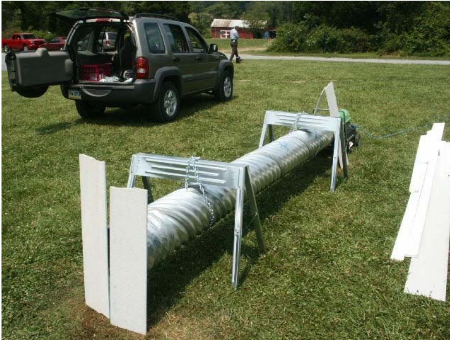
Pg 2-Culvert Heat Forming
