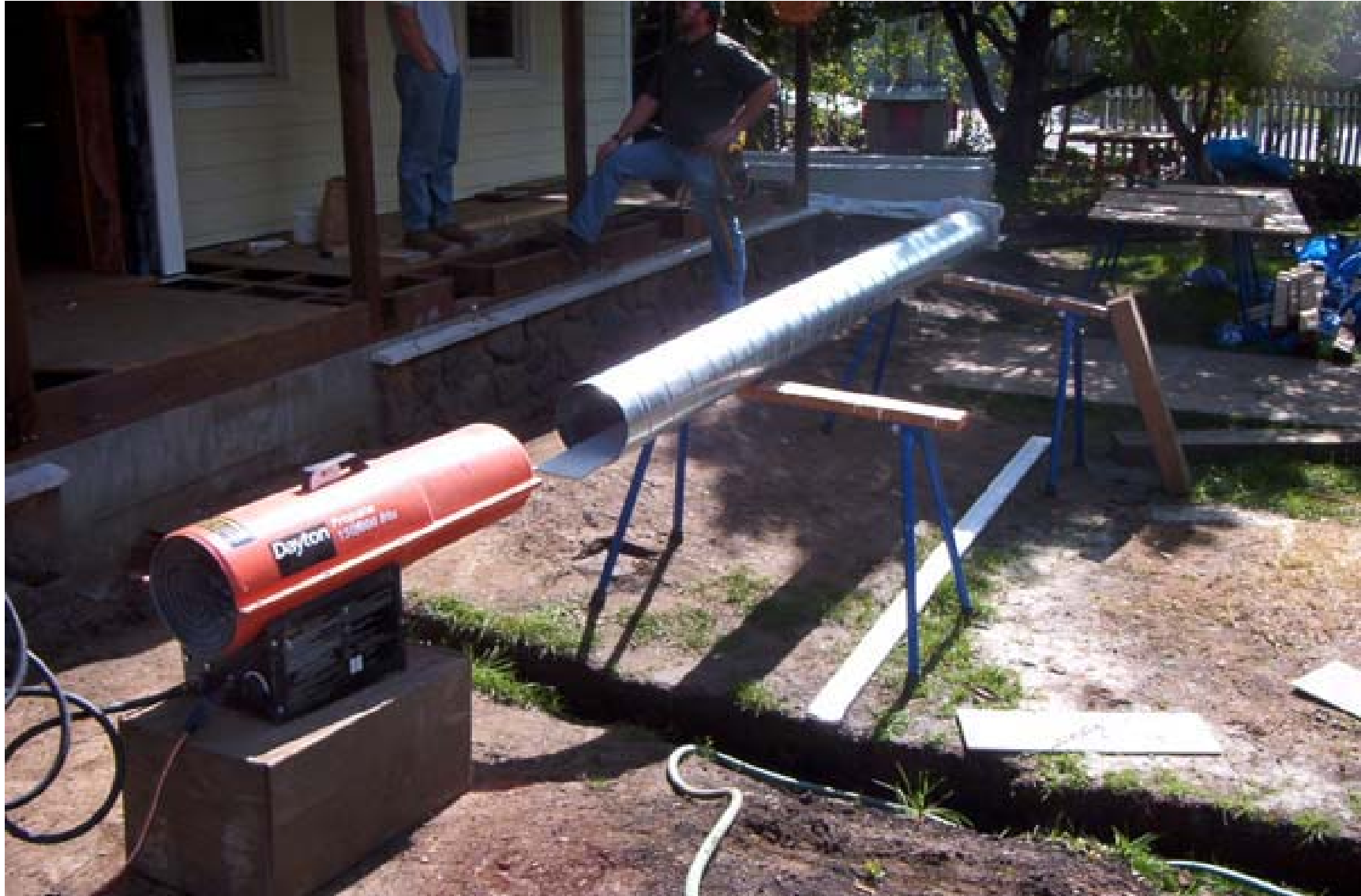
Pg 3-Culvert Heat Forming
