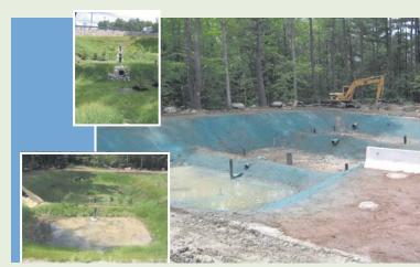
The fully vegetated gravel wetland [left top & bottom] exhibits excellent pollutant removal, provides subsurface anaerobic treatment, attenuates peak flow, and reduces flow volume. [Right] The gravel wetland's forebay and retention cells just after installation.
